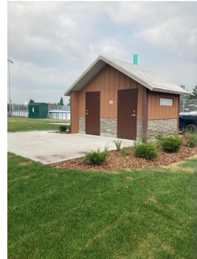
Outdoor Multi-Sport Recreational Facility Washrooms & Landscaping
